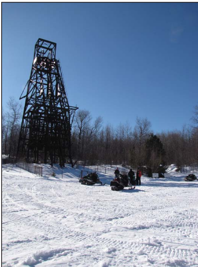
(Courtesy of Hurley Chamber of Commerce) The Plummer Mine headframe stands today as a reminder of our iron heritage. This is the last remaining headframe in the state of Wisconsin.
