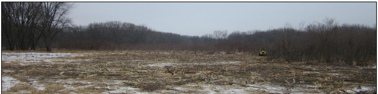
Brush Work Being Conducted in Spoehrs Marsh during January of 2018
