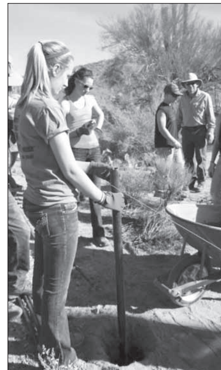
Leveling and setting posts for perimeter fence
